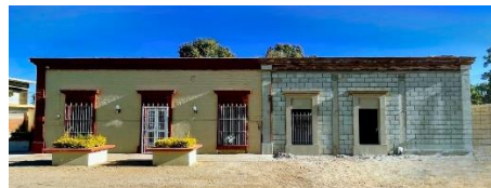
Construction in Alhuey
